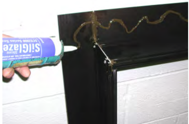
APPLY CAULK TO INSIDE LEG OF PANNING
