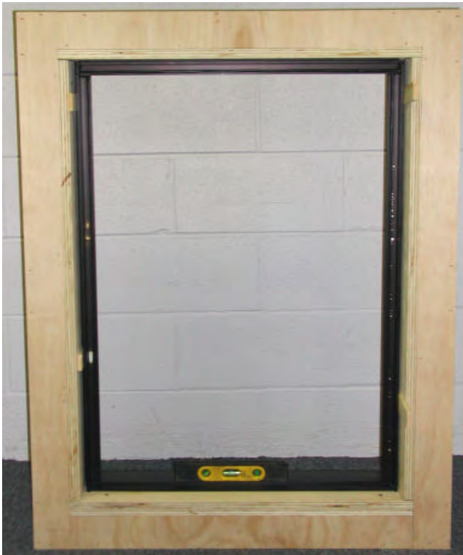
SLIDE PANNING INTO OPENING SHIM AND LEVEL
