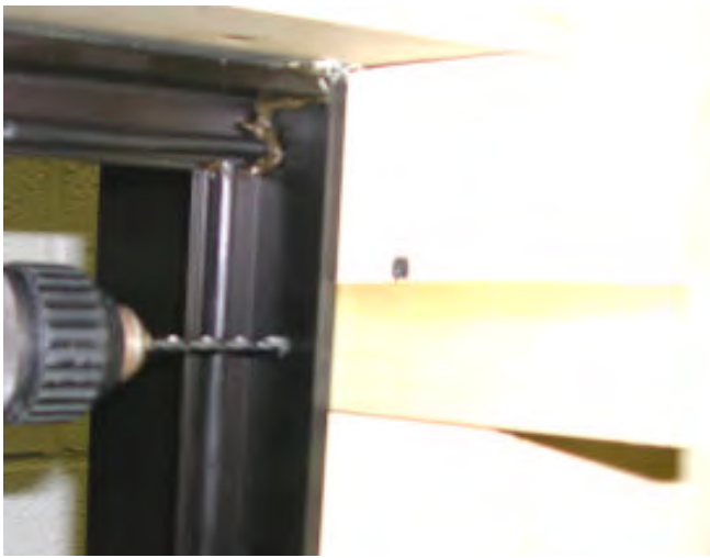
PREDRILL AND APPLY ANCHORS
