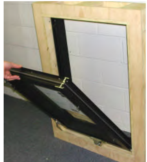
TILT WINDOW IN FROM INTERIOR
