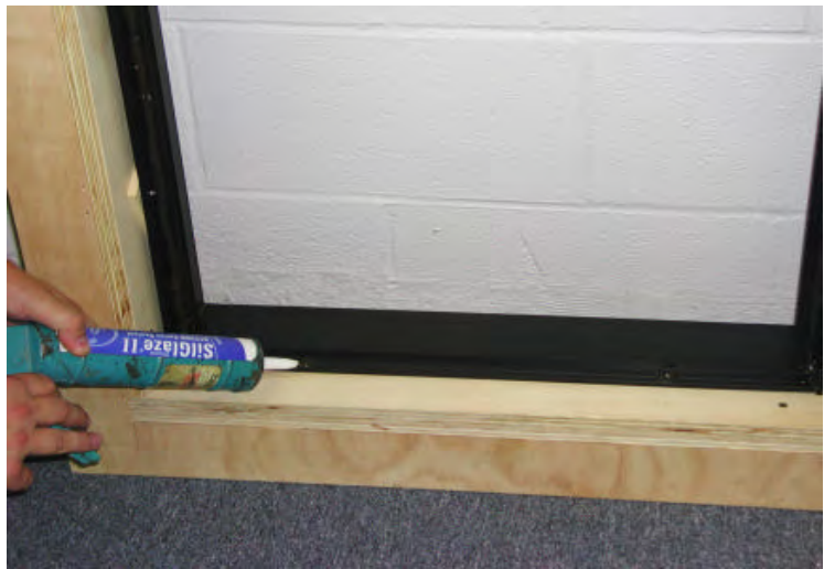
APPLY CAULK OVER ALL FASTENERS
