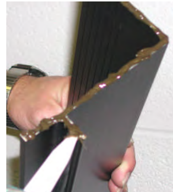
CAULK ENDS OF PANNING HEAD
