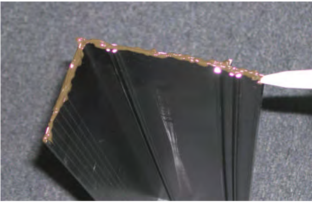
APPLY BEAD OF CAULK TO FULL SURFACE OF SILL ENDS
