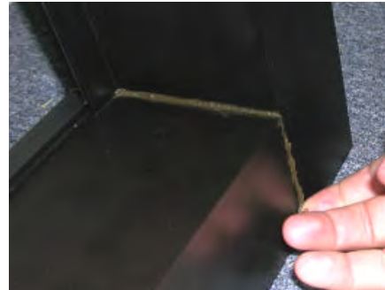
CAULK AND SMOOTH EXTERIOR SURFACE OF PANNING
